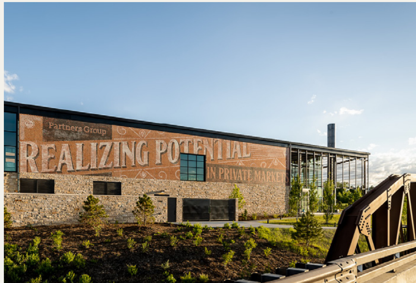
Partners Group campus | Denver, USA
